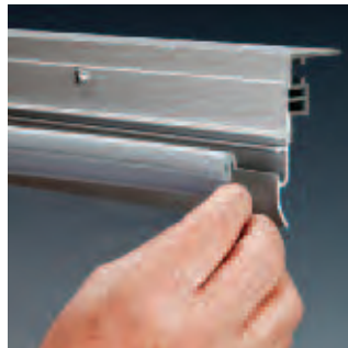
2. Unroll software panels and hook into place.
