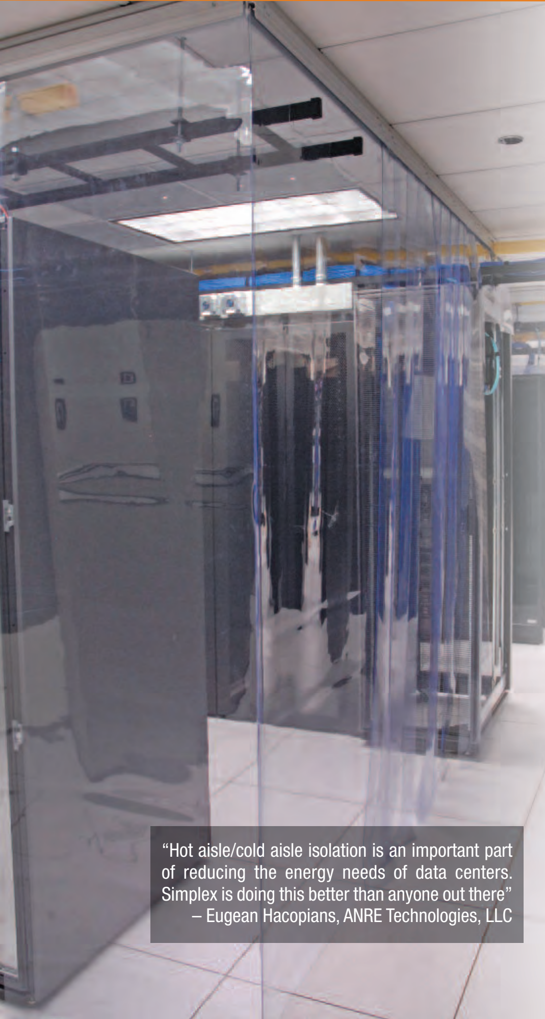
Curtains – Specify full length ceiling-to-floor curtains. Custom lengths for above-the-rack installations can be specified to accommodate racks of varying heights and widths, and from different manufacturers.
